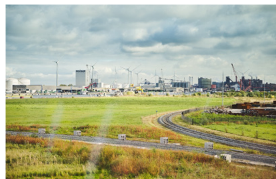
New ring railway in the port of Gent (North Sea Port).
