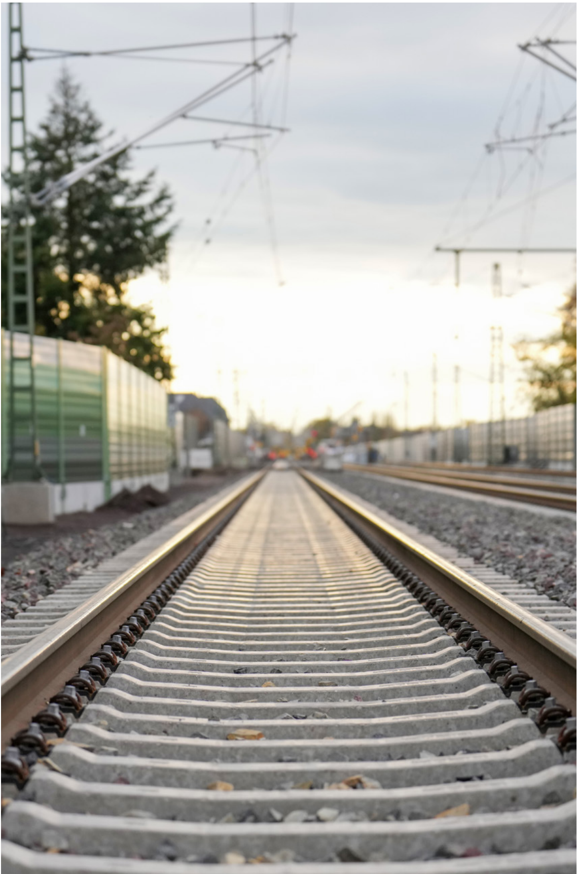
The line between Frankfurt and Darmstadt shortly before reopening in December 2024.
