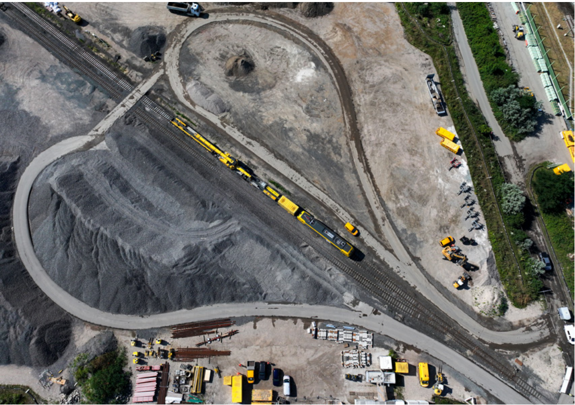
Aerial view of the general refurbishment of the Riedbahn in summer 2024.
