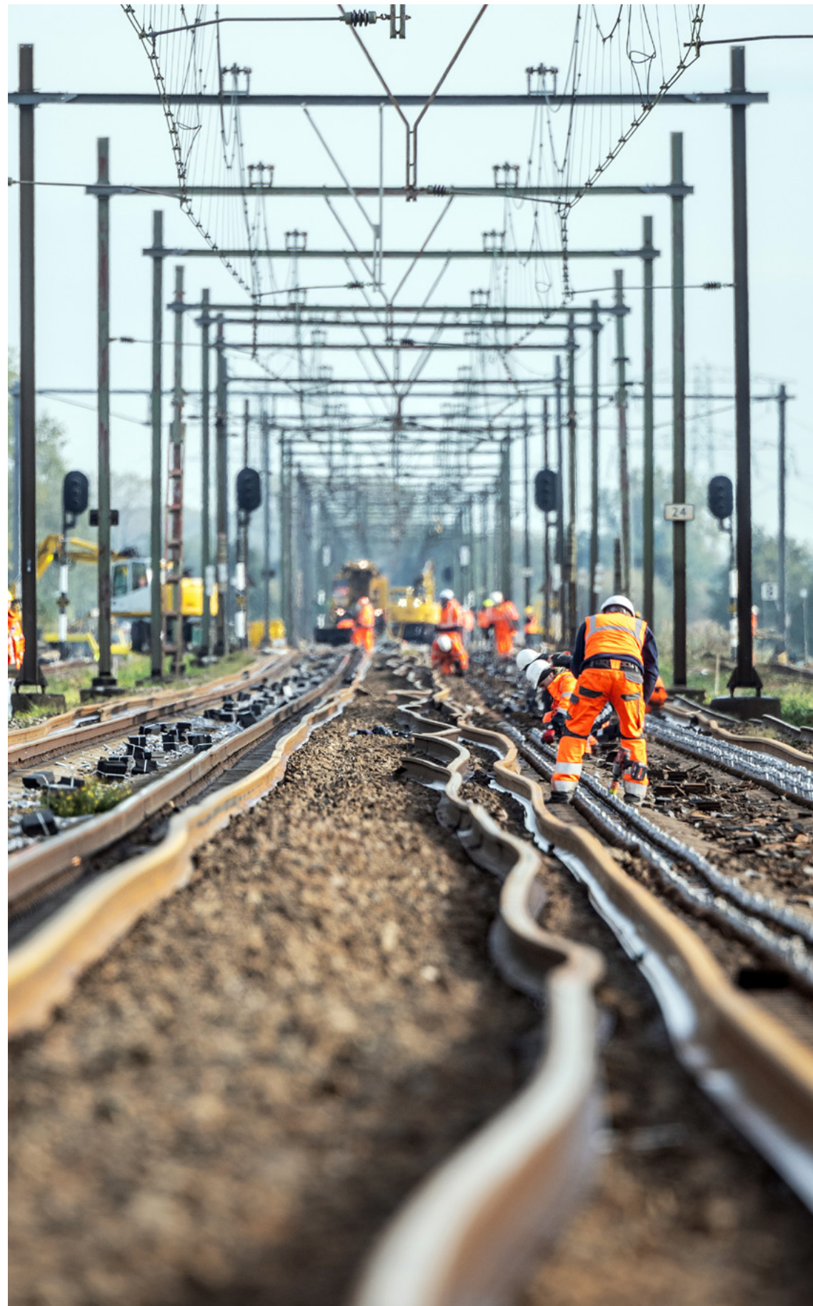
Rail infrastructure personnel operating in the Netherlands.
