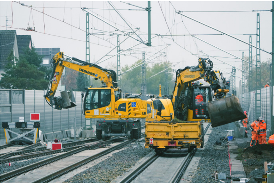
Construction works as part of the general renovation of the Riedbahn in September 2024.
