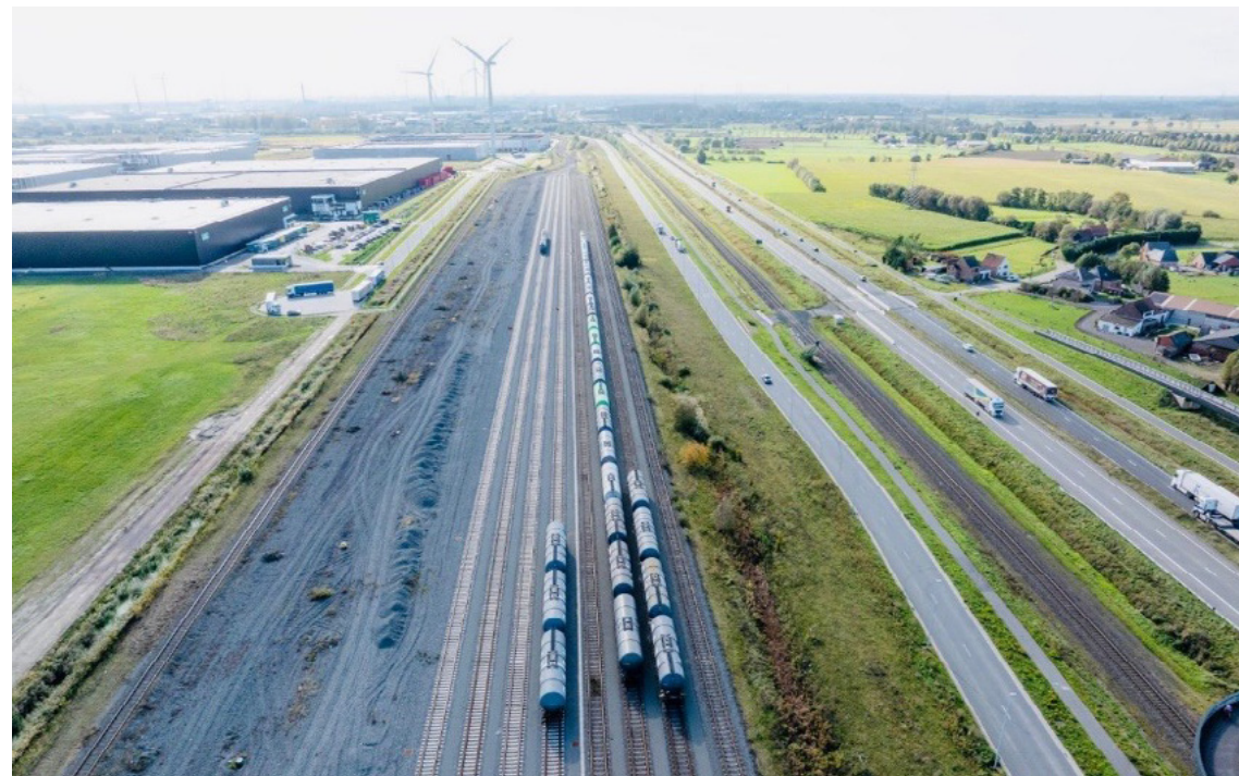
Fan of sidings "Zandeken", where in May 2023 – 4 additional long tracks were put into service.
