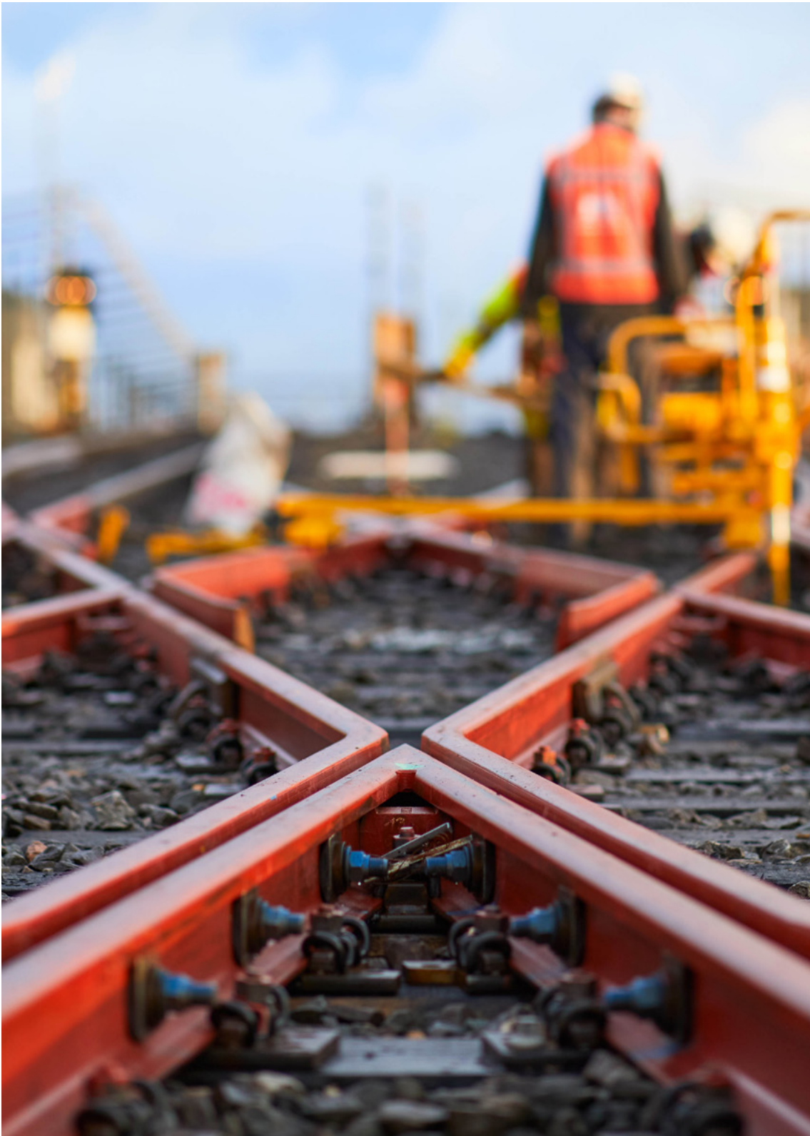
Emergency maintenance on a special rail switch at the Kijfhoek marshalling yard.
