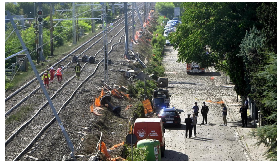
Repairing the tracks damaged by a derailment between Parma and Sant'Ilario.
