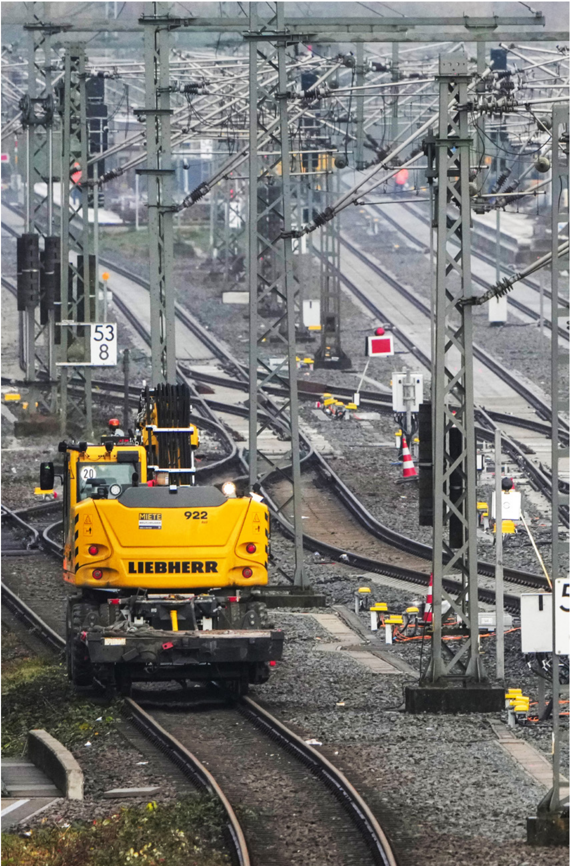
Construction works on the Riedbahn in autumn 2024.
